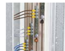
Modular circuit breakers connection bar
