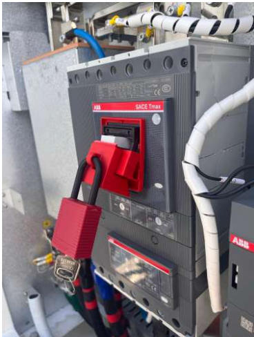
Figure 24. Breaker Unlock
