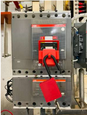
Figure 25. Lock Removal
