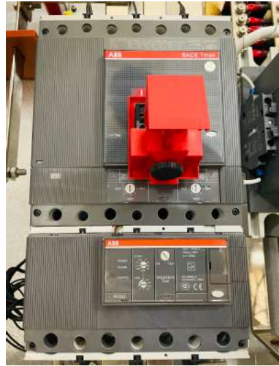
Figure 27. Remove Lock Flap
